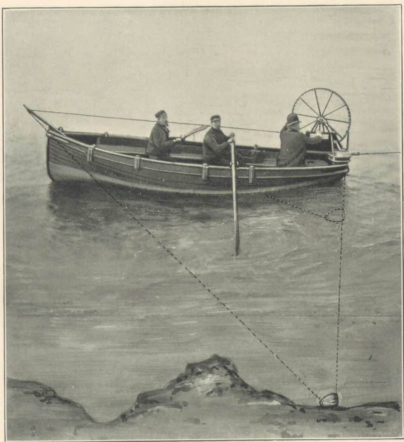
FIG. 42.—Sutcliffe's Sounding Apparatus.
