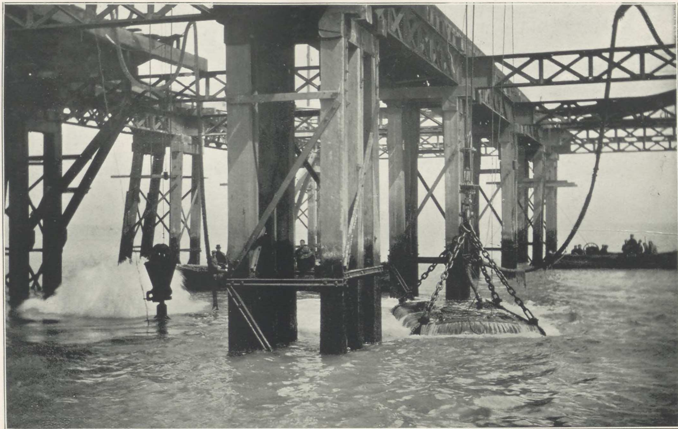
FIG. 56.—Submersion of Diving Bells at Folkestone Harbour Extension Works.
