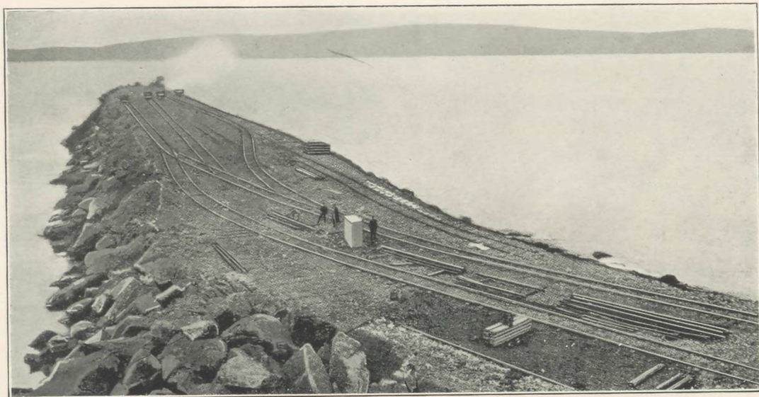
FIG. 85.—Fishguard Breakwater in course of construction.
