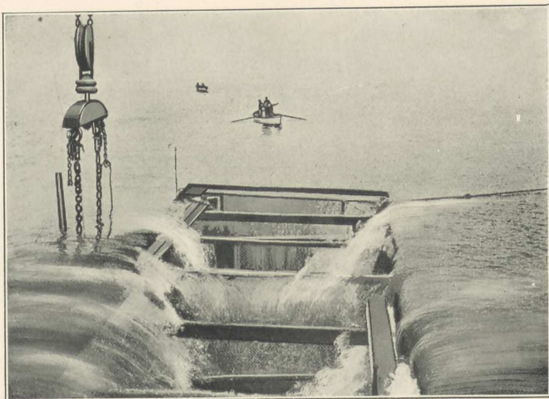
FIG. 151.—Sinking a Caisson at Zeebrugge Harbour Works.
