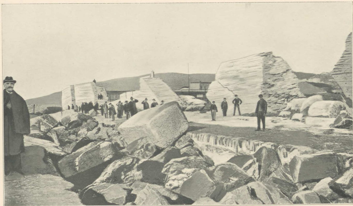
FIG. 113.—View of Genoa Breakwater after Storm of 1898.
