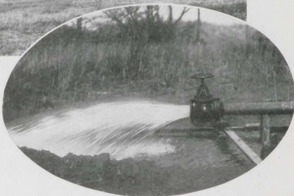
At the time of publishing this bulletin, Sullivan Air Lifts are being installed at the Municipal Water Works, Zanesville, Ohio. There will be 20 wells, drawing their supply from the Muskingum River. The cuts show the well drills at work, and a completed well being "back-blown."
