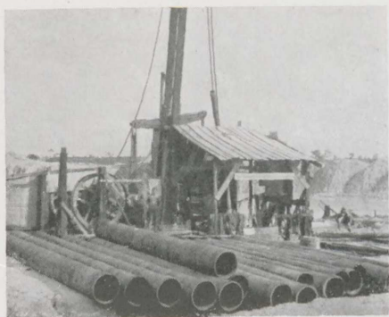
Drilling No. 9 Well, 16-in. in diameter, for Prairie Pebble Phosphate Co., Southard Contracting Company, Contractors
