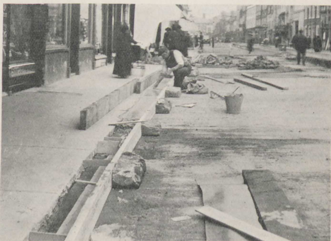
FIG. 8.—Concrete road in Northbrook Street, Newbury. The kerb is here seen under construction. In the foreground the strip of tarred paper will be observed lying in the bottom of the trench. The form is kept in position by spacers on the inside and blocks of stone on the outside.
