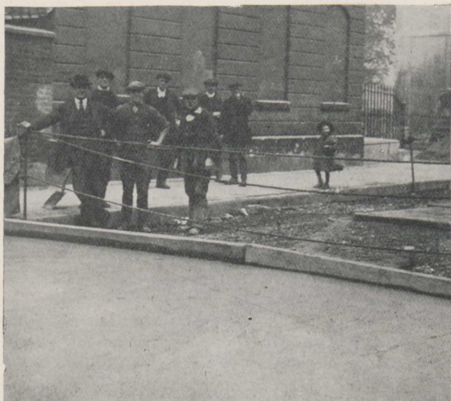
FIG. 1.—Concrete road in Brockham Street, Southwark. The end of a day's work. Note the planks by means of which the vertical edge is formed.
