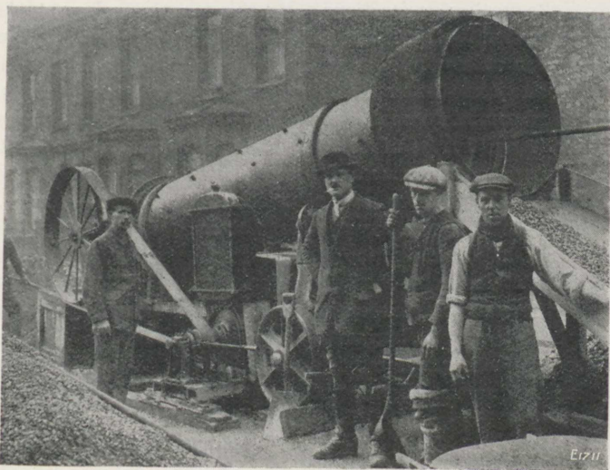
FIG. 95.—Baxter's Ballast-washing and Grading Machine, fitted with petrol motor. The machine, which is taken from street to street as required and connected to the nearest hydrant, was used by the Borough Council of Southwark for washing and grading the material from the old macadam roads.
