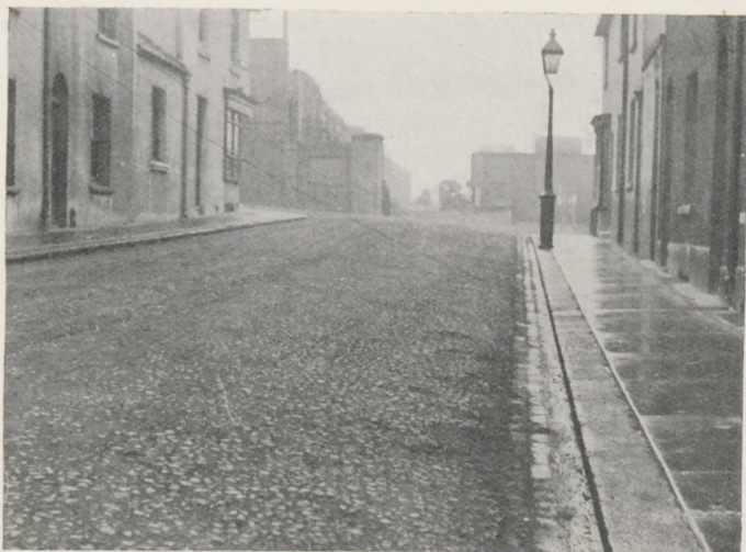
FIG. 121.—Concrete kerb and pitcher, and cement paving laid in 1878, in Brighton.
