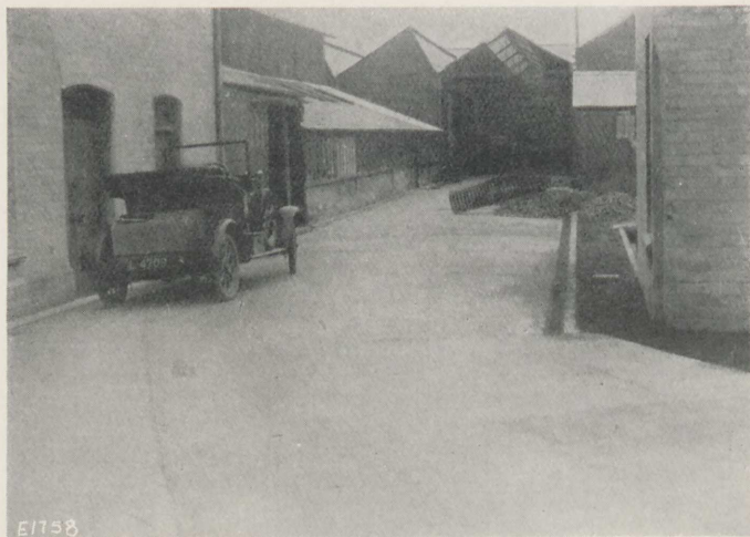
FIG. 65.—Road for Messrs. Lewis & Tylor, Ltd., Cardiff, laid May, 1920. Length, 164 ft.; width, 16 ft. Traffic: Motor lorries.
