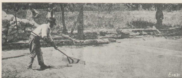
FIG. 111.—Use of Lute to place Concrete.
