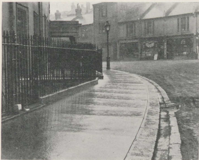
FIG. 122.—Concrete kerb laid in 1881 (and cement paving laid later), in Brighton.
