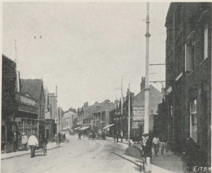
FIG. 39.—Bridge Street, Taunton, laid June, 1920. Surveyor, Mr. D. Edwards. Length, 500 yds.; width, 13 ft. 6 in. Traffic very heavy.
