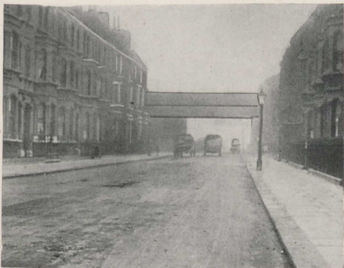
FIG. 2.—Concrete road in Steedman Street, Southwark. This thoroughfare has been open to traffic since August, 1919. Although the photograph was taken soon after a heavy shower of rain, it will be noticed that, with the exception of a few damp patches, the road is already dry.
