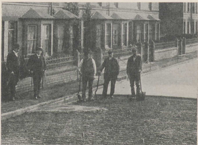
FIG. 9.—Showing metal reinforcement and the placing of the surface concrete, Roberts Lane, Chester.
