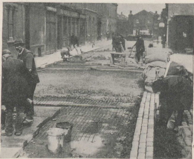
FIG. 4.—Concrete road under construction in New King Street, Deptford. The reinforcement for the lower course, stretched over a 2 inch plank in the foreground.
