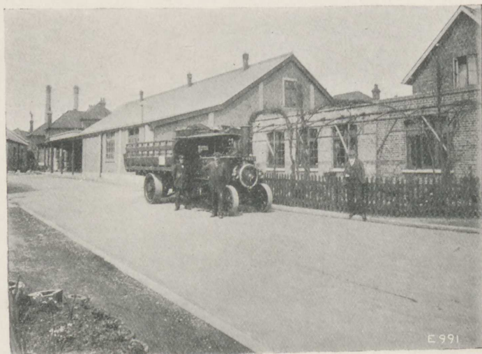
FIG. 48.—Reinforced concrete road at the works of Messrs. Joseph Baker, Sons & Perkins, Willesden Junction.
