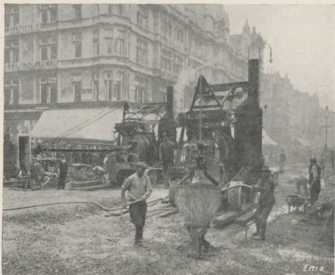
FIG. 114.—The Milwaukee Paver, showing method of discharging.
