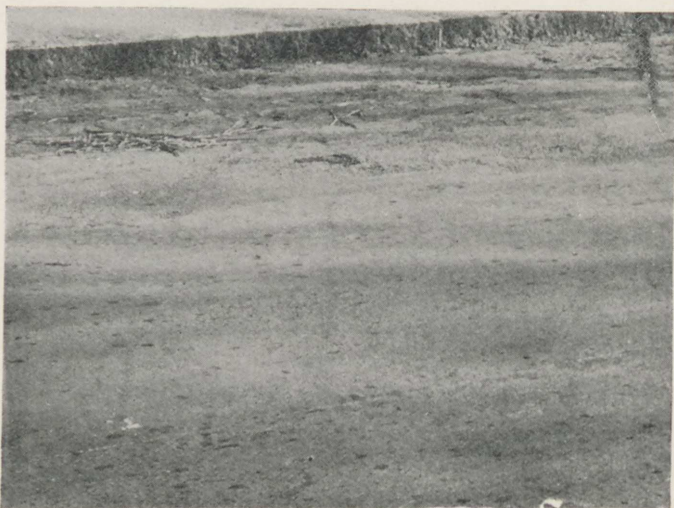
FIG. 33.—A close view of the surface of one of the bays of good concrete, which shows how level this remains after well over 5 years' wear. The half of the road which was laid 6:1 is in the background, and the contrast between the two halves is very noticeable in the photograph.
