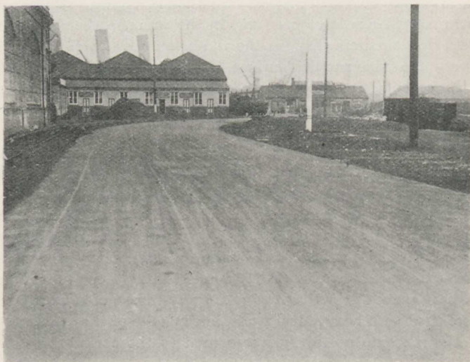
FIG. 29.—Reinforced concrete Dock Road, Southampton, for London and South-Western Railway.
