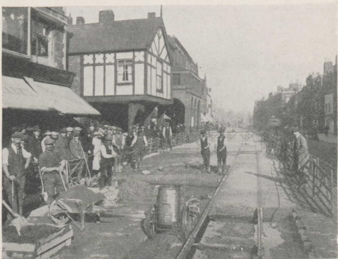
FIG. 12.—Road in course of construction, Foregate Street, Chester.
