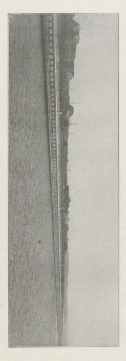
the harbour deepened. An examination of the bottom showed that not until reaching the depth of 60 to 70 feet a foundation could be in any measure secure. Above these depths the extensive layers consisted of a soft, sliding mass.
