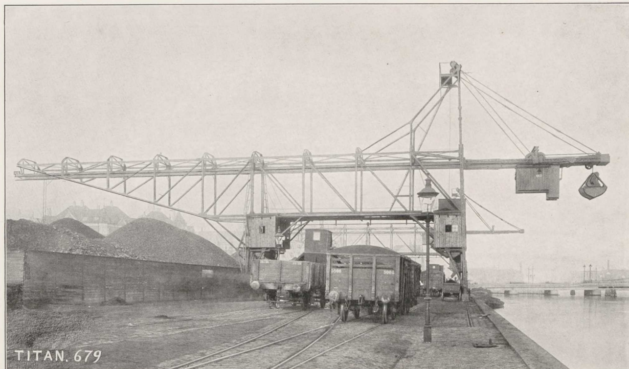
Coal discharging crane with 2m 3 grab. Capacity 90 tons per hour.
