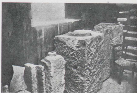
Roman Water Pipes made of Bored-out Blocks of Stone
