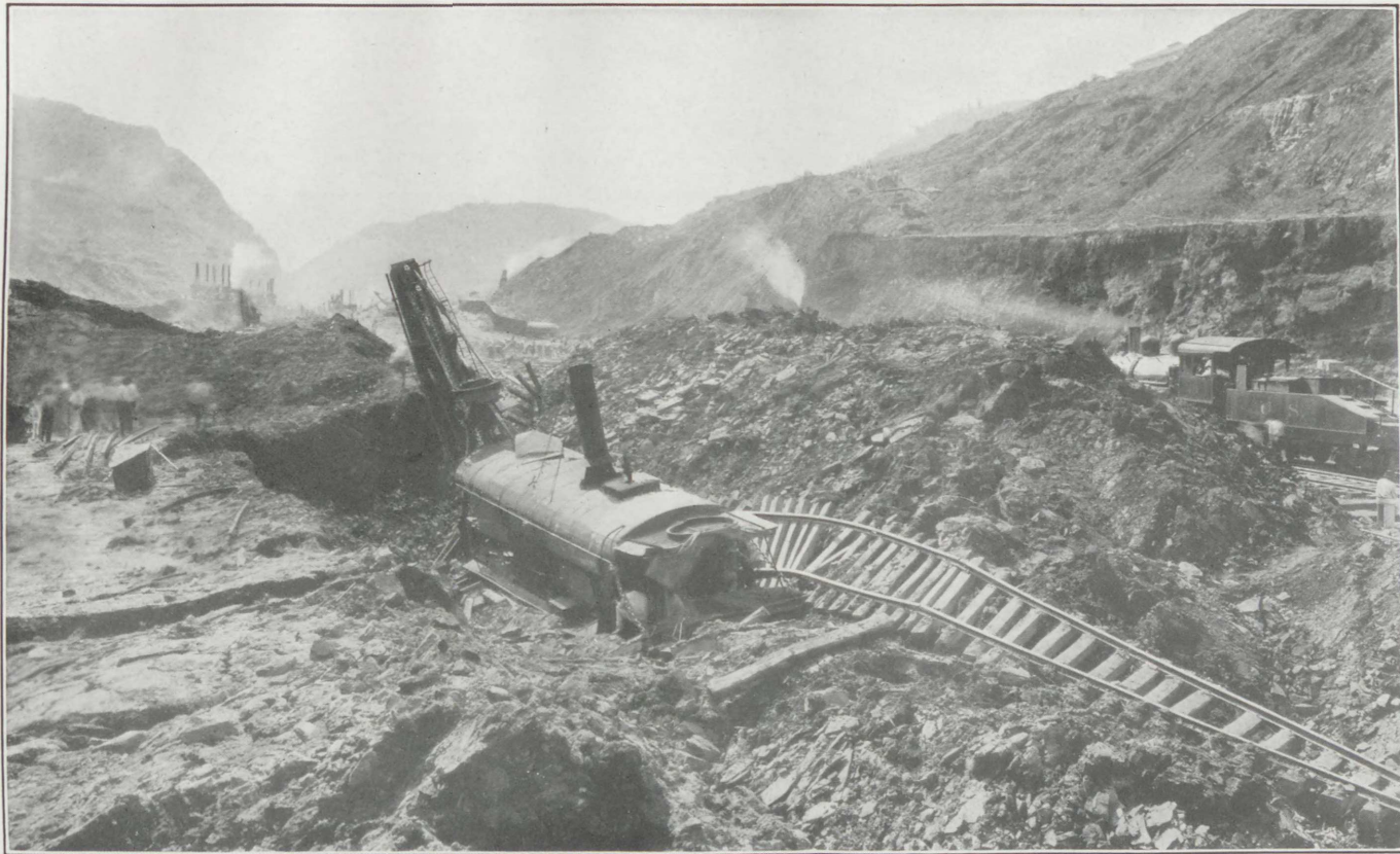
BULGING OF ROCKS IN BOTTOM OF CULEBRA CUT, CULEBRA, IN FRONT OF LARGE BREAK OR DEFORMATION SLIDE IN EAST BANK BETWEEN STATIONS 1746 TO 1758.
