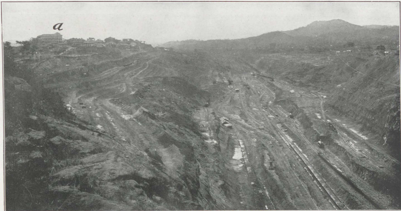
TERRACING ON BOTH SIDES OF CULEBRA CUT, NEAR CULEBRA, TO RELIEVE STRAINED CONDITION OF THE SLOPES. VIEW TAKEN FROM CONTRACTORS HILL, LOOKING NORTH.
