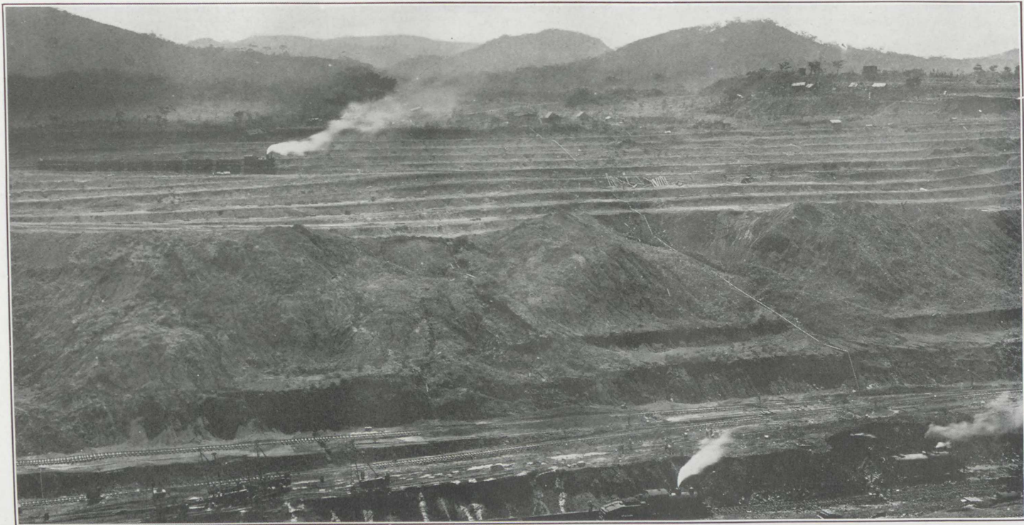
TERRACING TO RELIEVE STRAINED CONDITIONS OF SLOPES, EAST SIDE OF CULEBRA CUT, STATIONS 1735 TO 1765.
