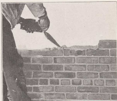
Fig. 33. — Handling mortar for two brick at one time on interior face tier.
