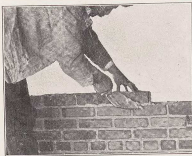
Fig. 32. — Cutting off mortar after brick is laid on interior face tier (here working left to right).
