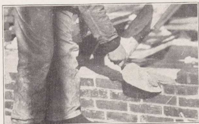
Fig. 30. — Cutting off mortar before brick is laid.
