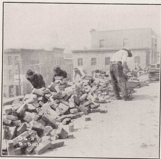
Fig. 9. — The usual method of providing the bricklayer with material.
