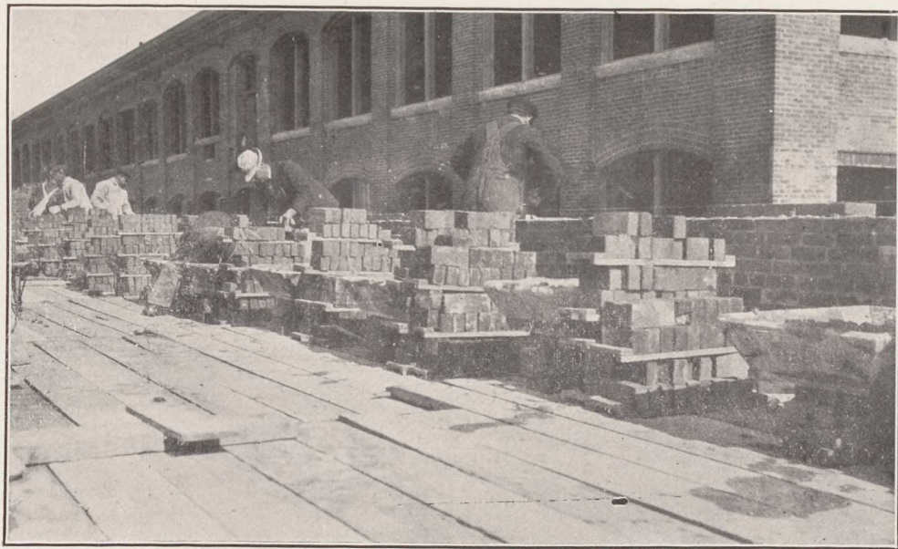
Fig. 11. — Standard practice of providing bricklayers with materials—raised mortar boxes and high piles of packs when the wall is waist high.
