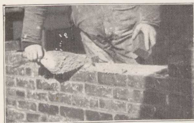
Fig. 26. — Buttering the end of the laid brick on the exterior face tier.
