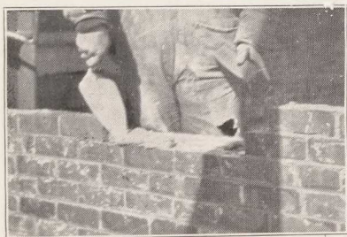
Fig. 24. — Spreading mortar on exterior face tier.
