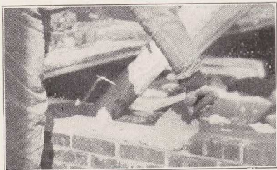
Fig. 28. — Throwing mortar on interior face tier.
