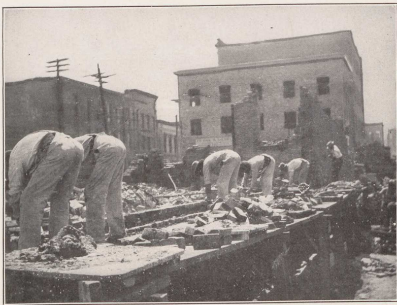
Fig. 23. — Common type of Trestle Horse Staging. Bricklayers cannot be expected to lay as many brick per day when working in this position as when standing up between a wall and a stock platform, each 2 ft. high.
