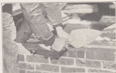
Fig. 31. — Tapping down brick after laying on interior face tier.
