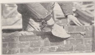
Fig. 38.—Working left to right.—Cutting off mortar after brick is laid on exterior face tier.
