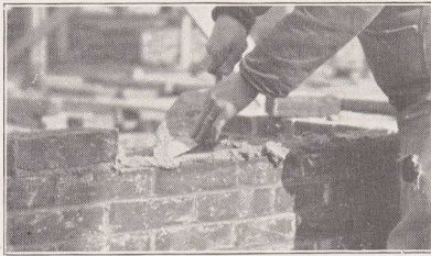
Fig. 40.—Working left to right.—Spreading mortar on the interior face tier.
