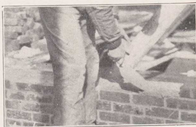
Fig. 29. — Spreading mortar on interior face tier.
