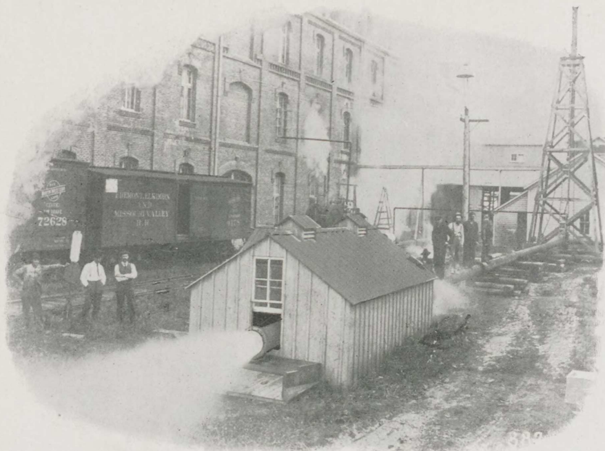
Air Lift Plant of the Standard Beet Sugar Co. at Ames, Neb. Capacity of 900 gallons a minute. Air pressure, 75 pounds. Lift, 200 feet.
