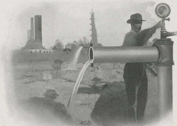
Wells at the Houston (Texas) Water Works, Showing the Flow Without the Application of Compressed Air.
