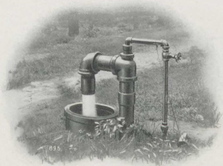
Discharge Pipe at One of the Wells. Air Lift Plant, Ravenna, O.
