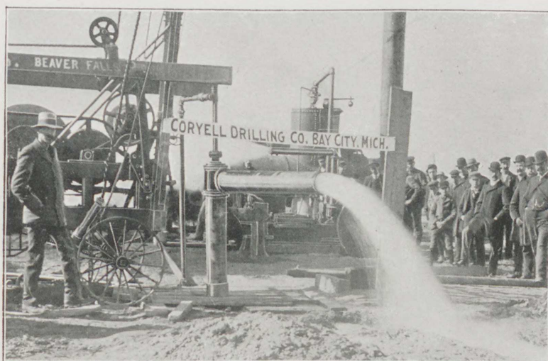
Testing an Air Lift Pump, Bad Axe, Mich.
