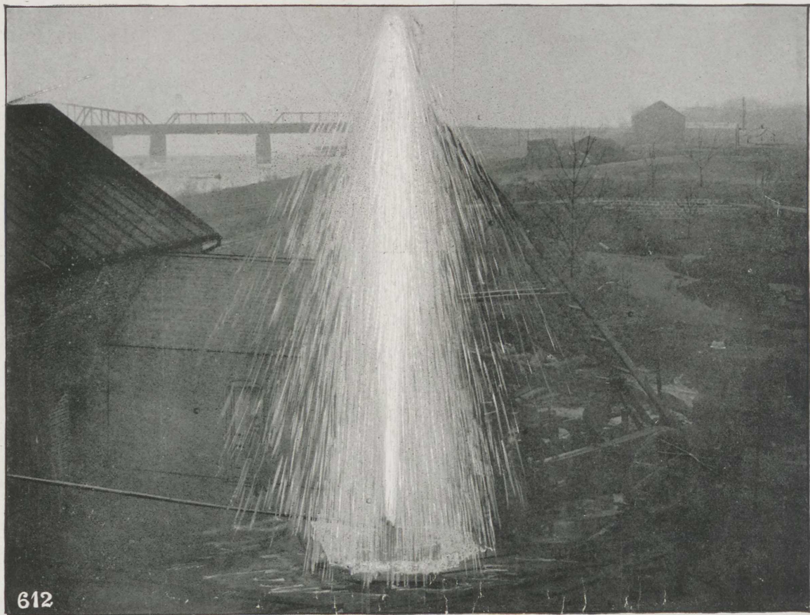
Air Lift at Fort Madison (Iowa) Water Works.
