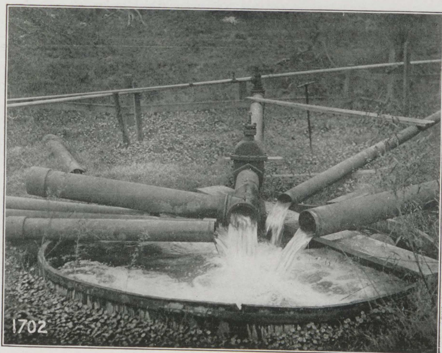
Water Discharge from Air Lift Wells at Houston, Texas.
