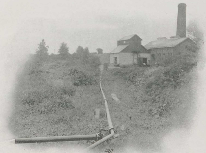
Compressor Power House for Operating an Air Lift.
