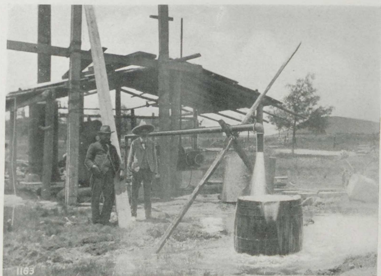
Discharge Pipe from an Air Lift at a Hacienda near Mexico City. The Compressor Plant, as Illustrated on the Opposite Page, is shown in the Background.
