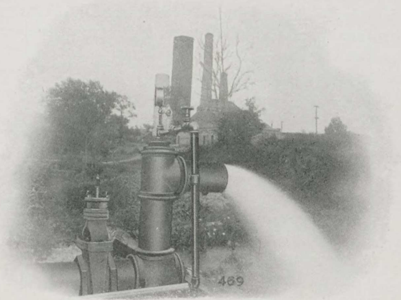
Wells at the Houston (Texas) Water Works, Showing Flow with the Application of Compressed Air.
