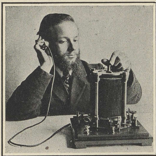
FIG. 97.—Bellini-Tosi radio-goniometer for directive wireless telegraphy.
